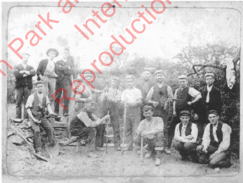
Digging the foundations of the Sunday School.
